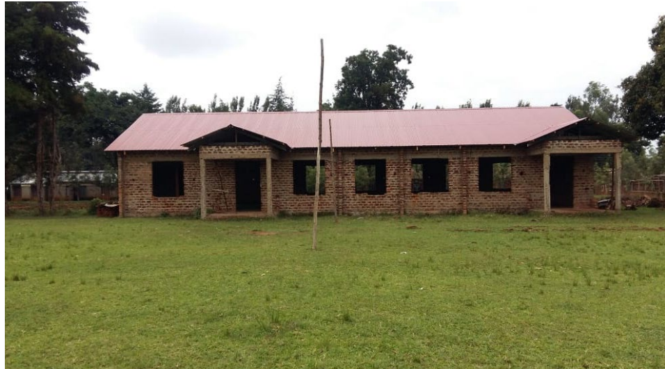
Construction of Musanda Sec. School dormitory
