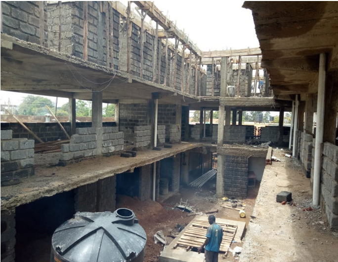
Construction of commercial building in Siaya Town
